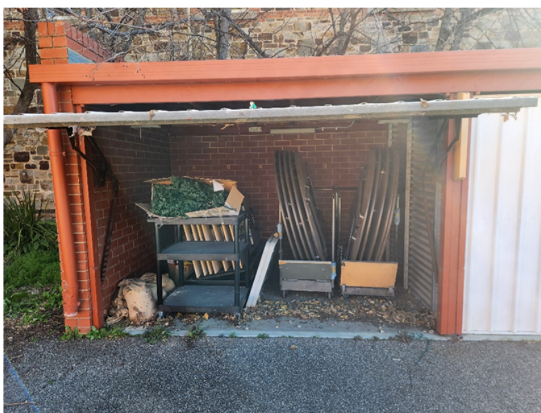
Figure 5: Storage sheds adjacent to the community centre – internal view
